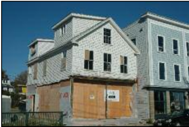
214-218 under construction and renovation. Renovations to 218 to the far right have been completed. Eventually a new building will be constructed to the left of 216 Main Street.
