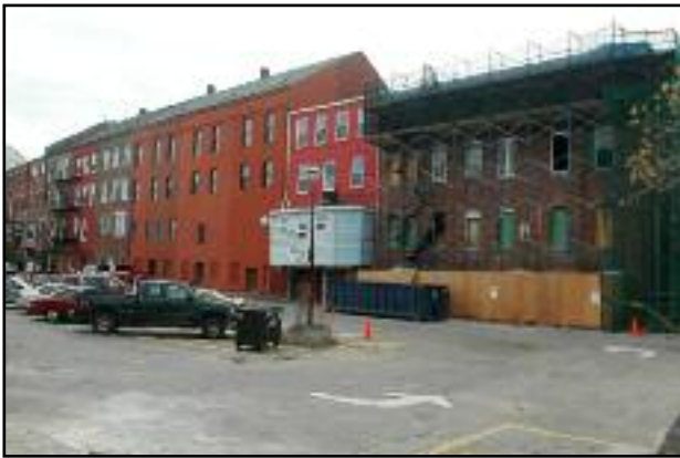
The back of 449 Main Street currently under renovation. This row of buildings makes up the Custom House Block and is an area envisioned with parking lot level access to commercial uses. 441 Main Street, the red building with the blue expansion has access to the Rockland Cafe.
