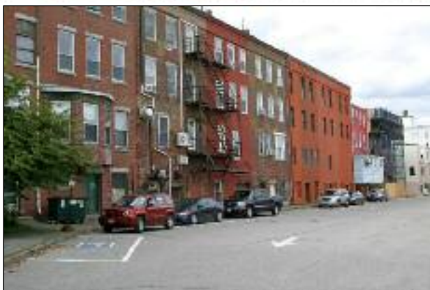
As additional development occurs in lower level of harbor side buildings, such as with the Custom House Block, more attention will have to be given to the management of parking to support revitalization efforts.
