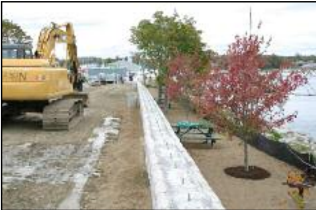
Work is completed on the Schooner parking area and adjacent park along the Wastewater Treatment Drive. This is an important construction of a section of the Trail, but the Harbor Trail will have to be carefully integrated into a sidewalk and open space system with the redevelopment of the Tillson District in order to create a strong connection to the existing Harbor Walk constructed by MBNA.
