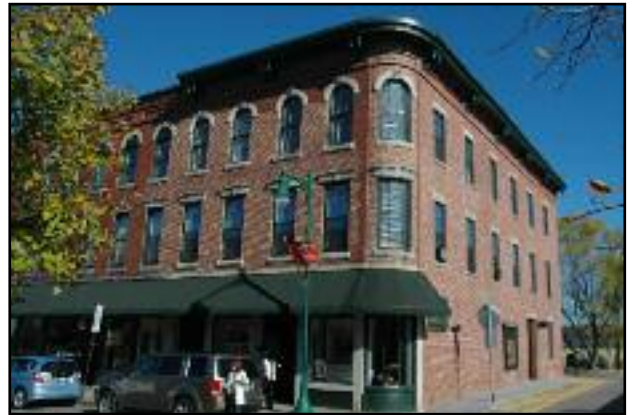
A Main Street building on a corner lot addressing both frontages with consistent, high quality materials and renovations.
