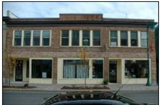
453 Main Street with recently renovated 1st and 2nd floors. This building frames the alley to the public parking lot behind the Custom House Building. The façade has been carefully restored and the proportions of the 1st floor and 2nd floor windows emphasize the traditional use of the 1st floor for commercial uses and the 2nd floor for commercial or residential uses. This image shows the completed Phase 1 streetscape improvements.
