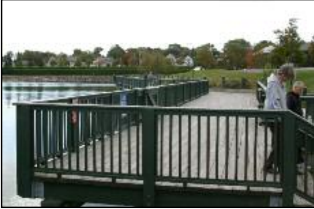
Existing Harbor Walk constructed by MBNA.
