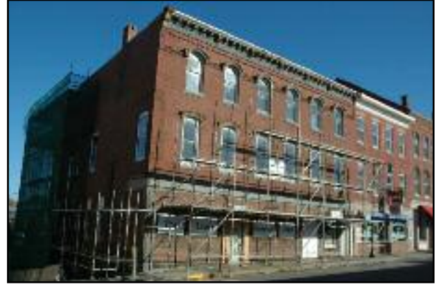
Front façade improvements to 449 Main Street. Also rear façade or harbor side improvements have been made as well as interior renovations.
